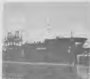
Part of the Pier Modernization Project is replacement of existing loading structure (left) by new loading facilities shown at right.
